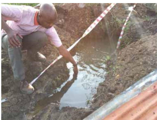
Figure 1.10.5 (above): An illegal connection that was left leaking at Phathane in uMfolozi Municipality
