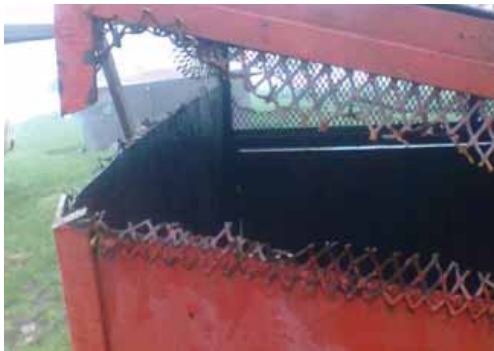
Figure 1.10.3: Cage cut to steal fuel in Machunwini in Nkandla
