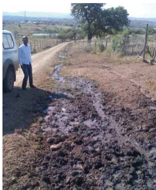
Figure 1.10.5 (above): An illegal connection that was left leaking at Phathane in uMfolozi Municipality
