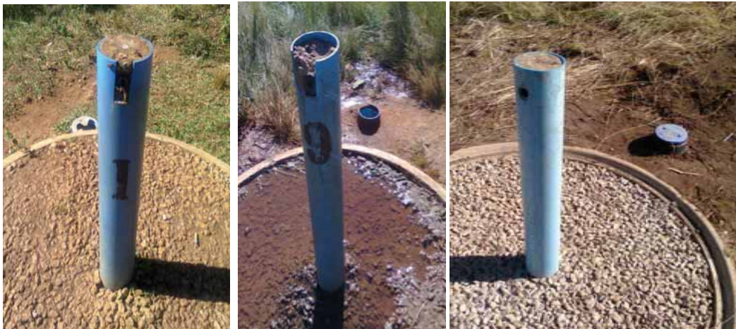
Figure 1.10.5: Taps stolen at Nkulisabantwana in uMlalazi with water usually left gushing out of standpipes for hours
